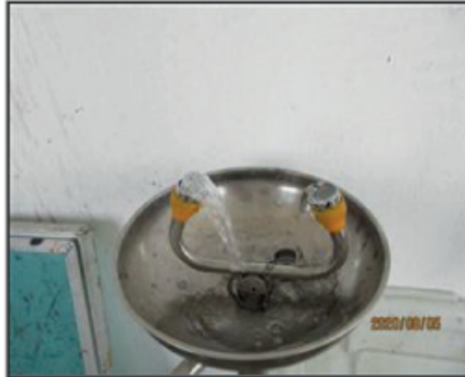
External photo(s) of the production unit(s) 7.7 Less water pressure of the eye wash facility.JPG
