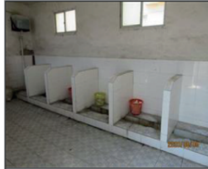
External photo(s) of the production unit(s) 7.22 No privacy door of toilet in production building.JPG
