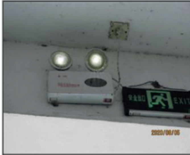
External photo(s) of the production unit(s) Emergency light test.JPG
