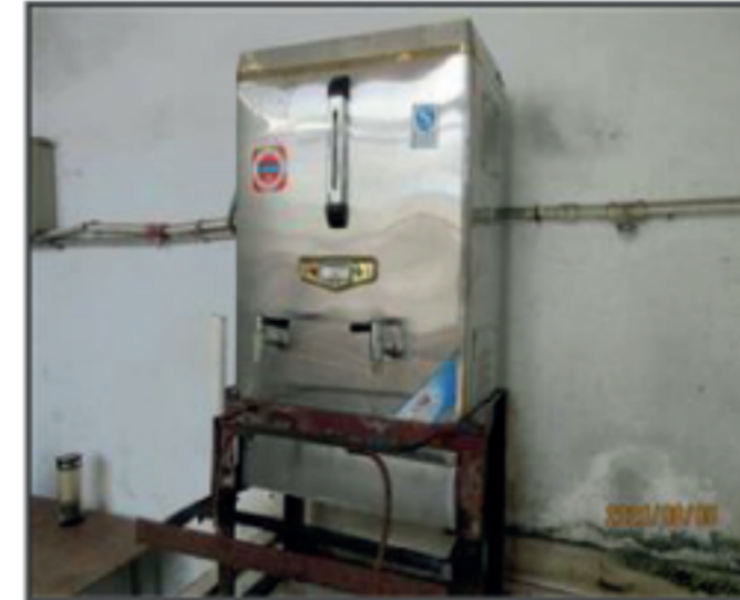
External photo(s) of the production unit(s) Drink water.JPG
